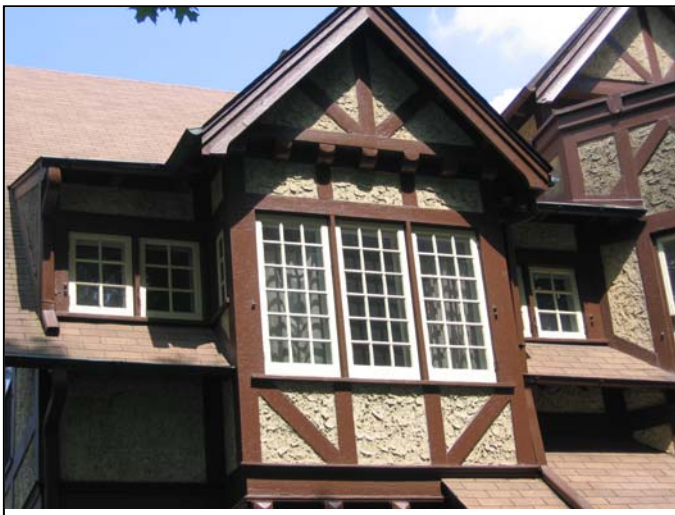
Historic, wood casement windows in the Wyncote Historic District.
