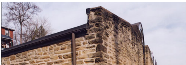
This shallow sloped roof terminates at a decorative parapet.
