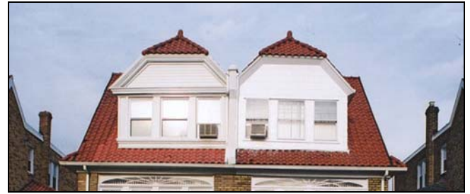
Paired jerkin roof dormers provide additional inhabitable space at the upper level and interrupt the unifying side gable roof of these twin residences.
