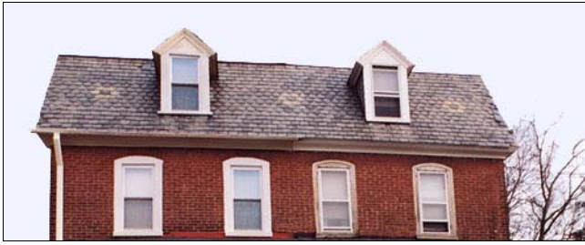
The banded slate shapes and the addition of a color pattern enhance this simple twin house.
