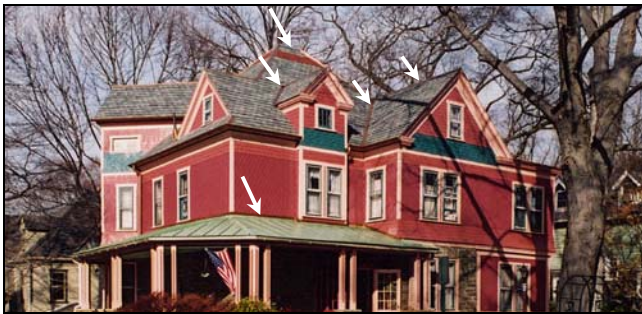
The arrows indicate typical flashing locations.
