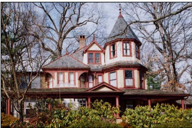
The dormers, tower and chimney punctuate this Victorian roof.
