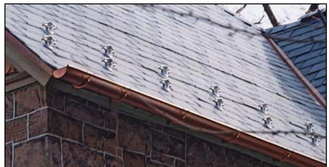
*Snow birds provide protection and a visual pattern at the edge of this roof. Note the half-round gutter installation.*
