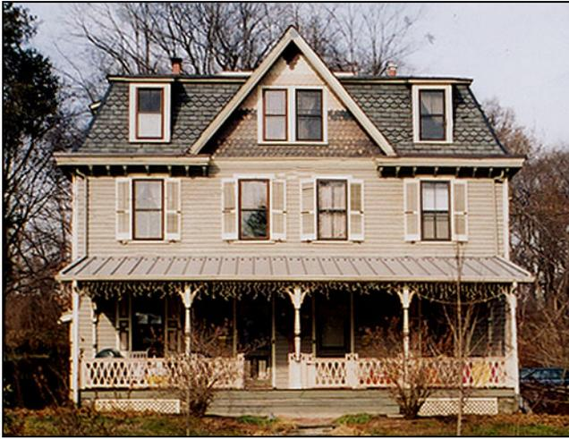
*The slates on this Mansard roof were replaced with dimensional asphalt shingles to replicate the color and pattern of the original.*
