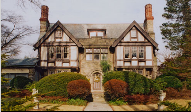
The pair of fluted gable end brick chimneys is a characteristic of the Tudor Revival style, as is the central shed roof dormer.
