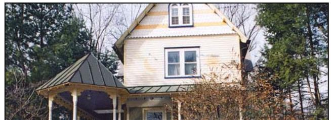
*Standing seam metal roofing can be found at steeply pitched roofs, while flat seam metal roofing is more typical at shallower roofs.*
