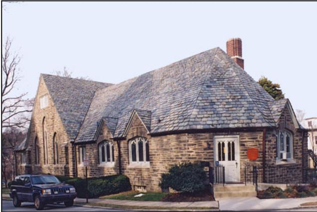
*The roof slates at this church are varied in color, size and thickness. Larger slates are located at the roof eaves with smaller slates at the ridge. This graduating pattern makes the roof appear visually larger. The gable dormers break up the continuous eave line.*
