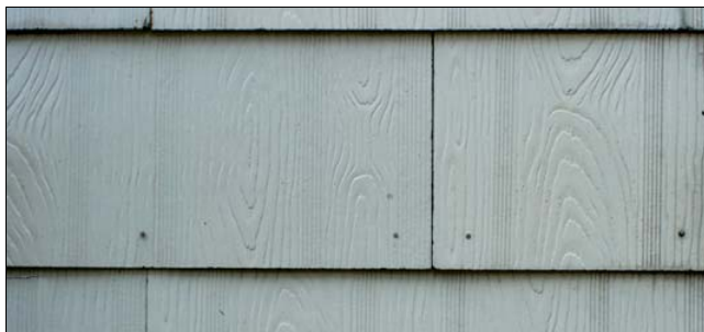
Asbestos siding is often embossed with a wood grain pattern. The removal of asbestos siding can be dangerous and should be undertaken by trained professionals.
