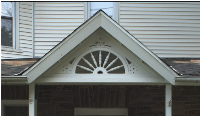
Although the walls of this residence were covered with artificial siding, the decorative wood pediment remains exposed to view.
