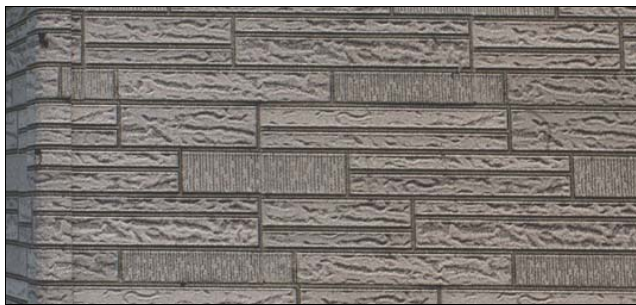
Asphalt siding often simulates brick or stone wall surfaces.
