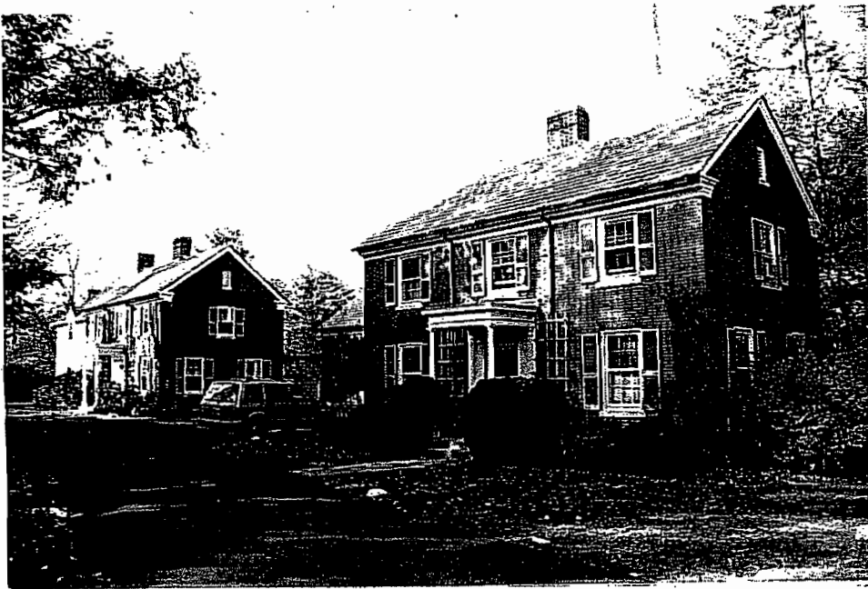
(5) View of the caretaker's houses. Note Colonial Revival details.
