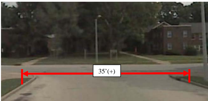
Wide Streets, no crosswalks ADA ramps not to current standards
