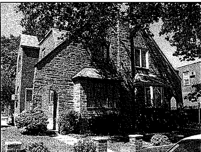
These semi-attached dwellings in the La Mott Historic District illustrate the role that windows play in the appearance of a building. The dwelling on the left has the original steel casement windows, whereas the one on the right has modern vinyl windows.
