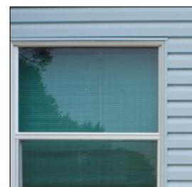
*The window frame has been completely covered with the vinyl siding. Without the frame, the visual dimensions of the window are changed and character of the building diminished.*
