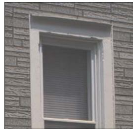
*The wood window frame remains exposed in spite of the application of asphalt siding. The exposed woodwork adds visual interest and is in keeping with the size and proportion of the window.*
